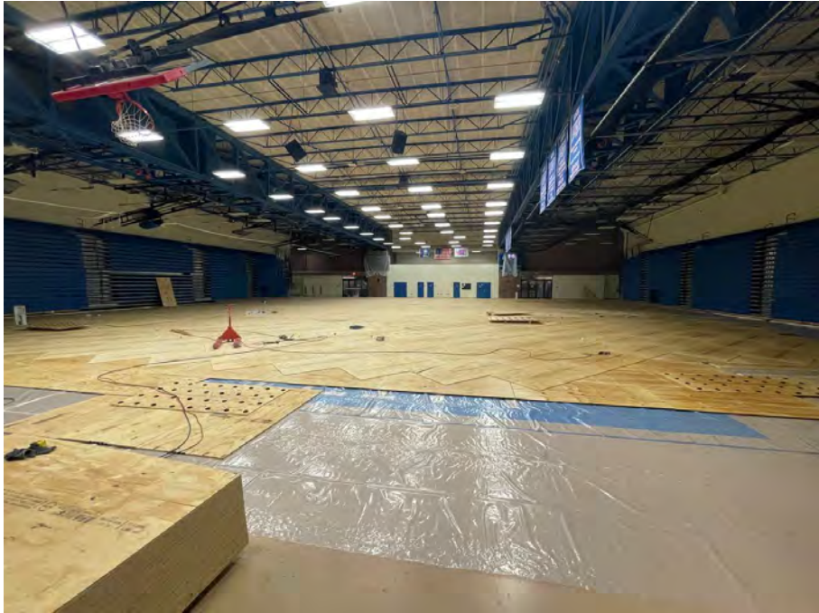
Field House Subfloor Installation:
