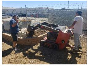
BEMT students Mauricio Ortiz and Alexis Cruz Gonzalez utilized the Toro Dingo Compact Equipment Loader. Students installed the retaining wall, backfilled with gravel for drainage, and placed topsoil for planting greenery as part of their Landscaping course.
