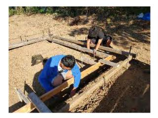
BEMT students used equipment to dig a training foundation, build concrete forms, and install/cut steel reinforcing bars.
