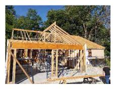
As part of the Carpentry Basics course in the BEMT Program, students built and installed all exterior walls, ceiling joist framing, and most the roof structure at the program's land bank house. Students learned to read span charts, cut rafters, and install stabilizing braces to the roof superstructure. The next step for student learning is installation of doors and windows to close the house to the weather.
