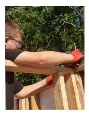
BEMT high school student Courtney Anderson installs framing nails to secure the exterior wall sheathing to the rim joist increasing the strength and rigidity of the structural members. Students have framed and stood all the exterior walls and interior walls at the BEMT Program's Land Bank House. BEMT students will begin to frame the ceiling and roof as part of their carpentry class.
