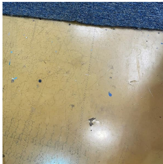
Photo 2: Room 3800 – View of observed gouges in exposed rubber flooring.
